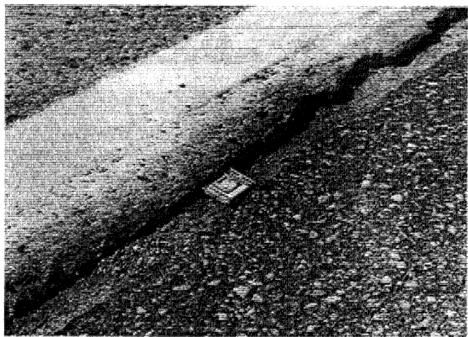
Figure D2 - Lane/Shoulder Separation
