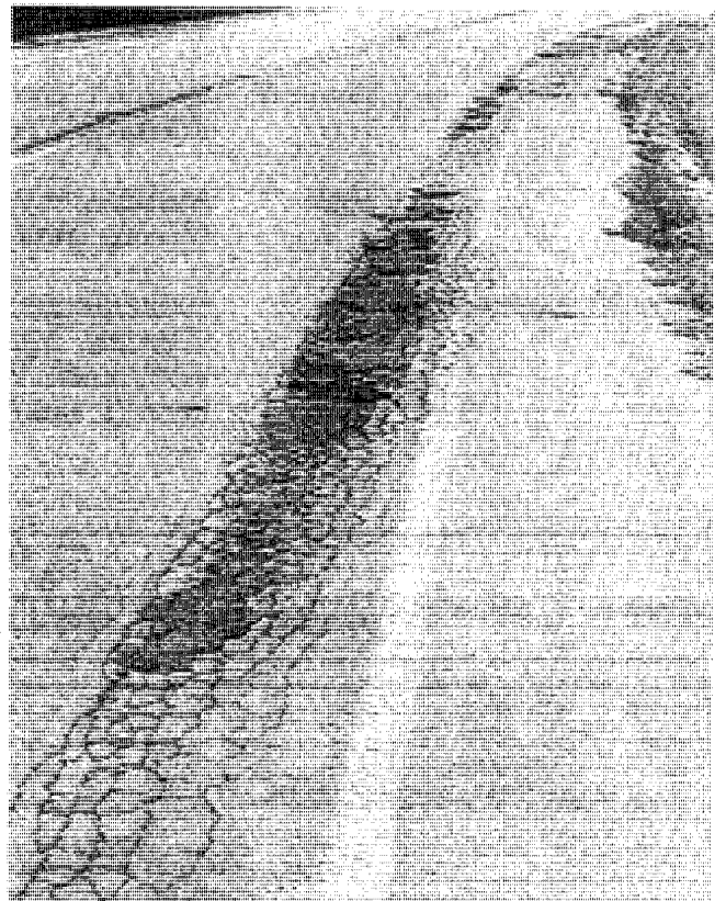
Figure C7 - Edge Cracking
