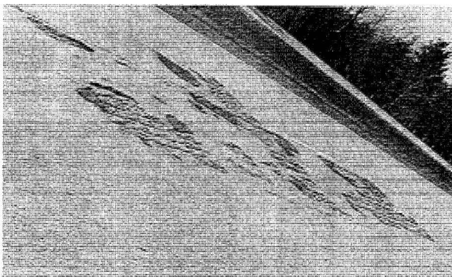
Figure B12 - Scaling Non-Joint Spalling
