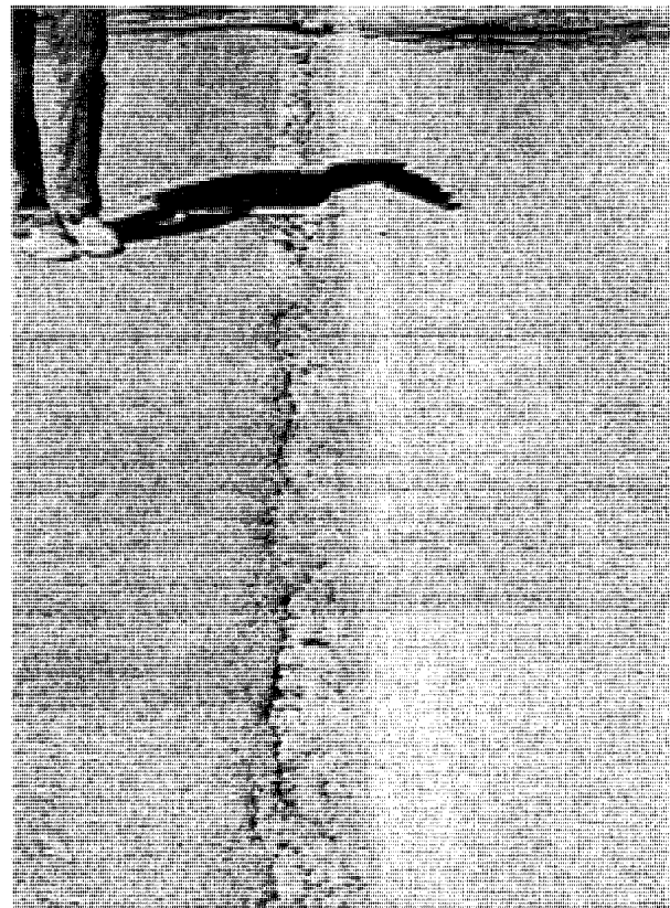
Figure C6 - Longitudinal Cracking
