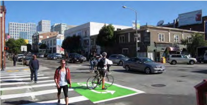
Two-stage turn queue boxes provide a holding area for bicyclists to queue, allowing them to cross an intersection in two stages in the San Francisco area. This crossing pattern is more comfortable, especially for less experienced bicyclists.
