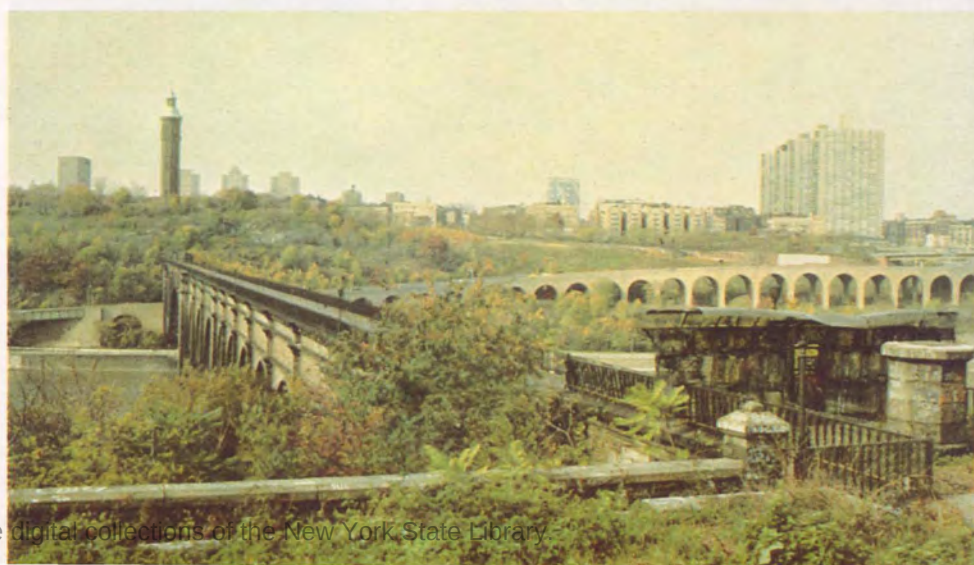
(Above) The Cornell or New Croton Dam is the largest masonry dam and spillway ever built. (Below) Highbridge, where the aqueduct crosses the Harlem River, has 15 semicircular arches.
