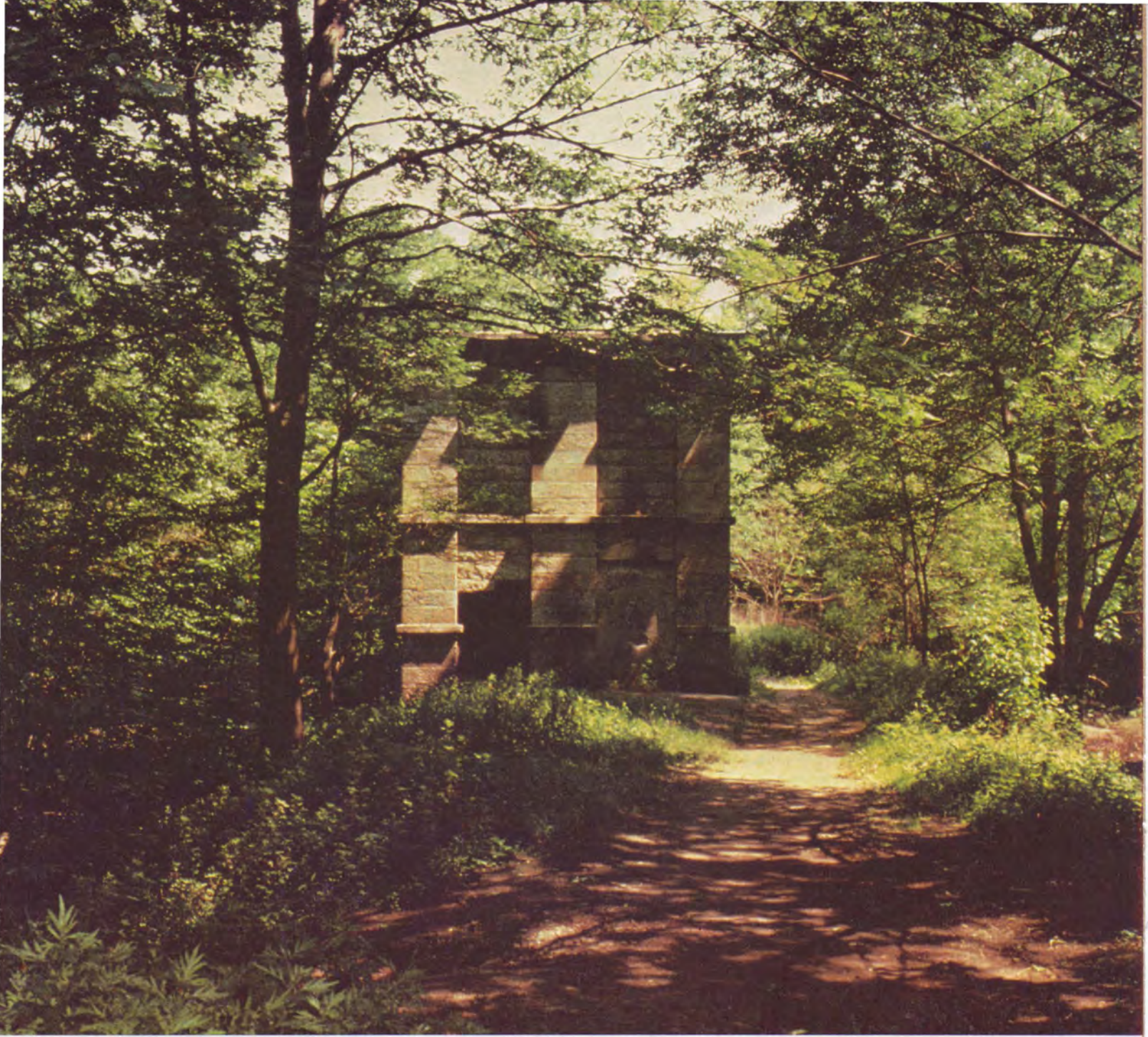
Gatehouse/blowout tower in Van Cortlandt Park, Bronx, N.Y.
