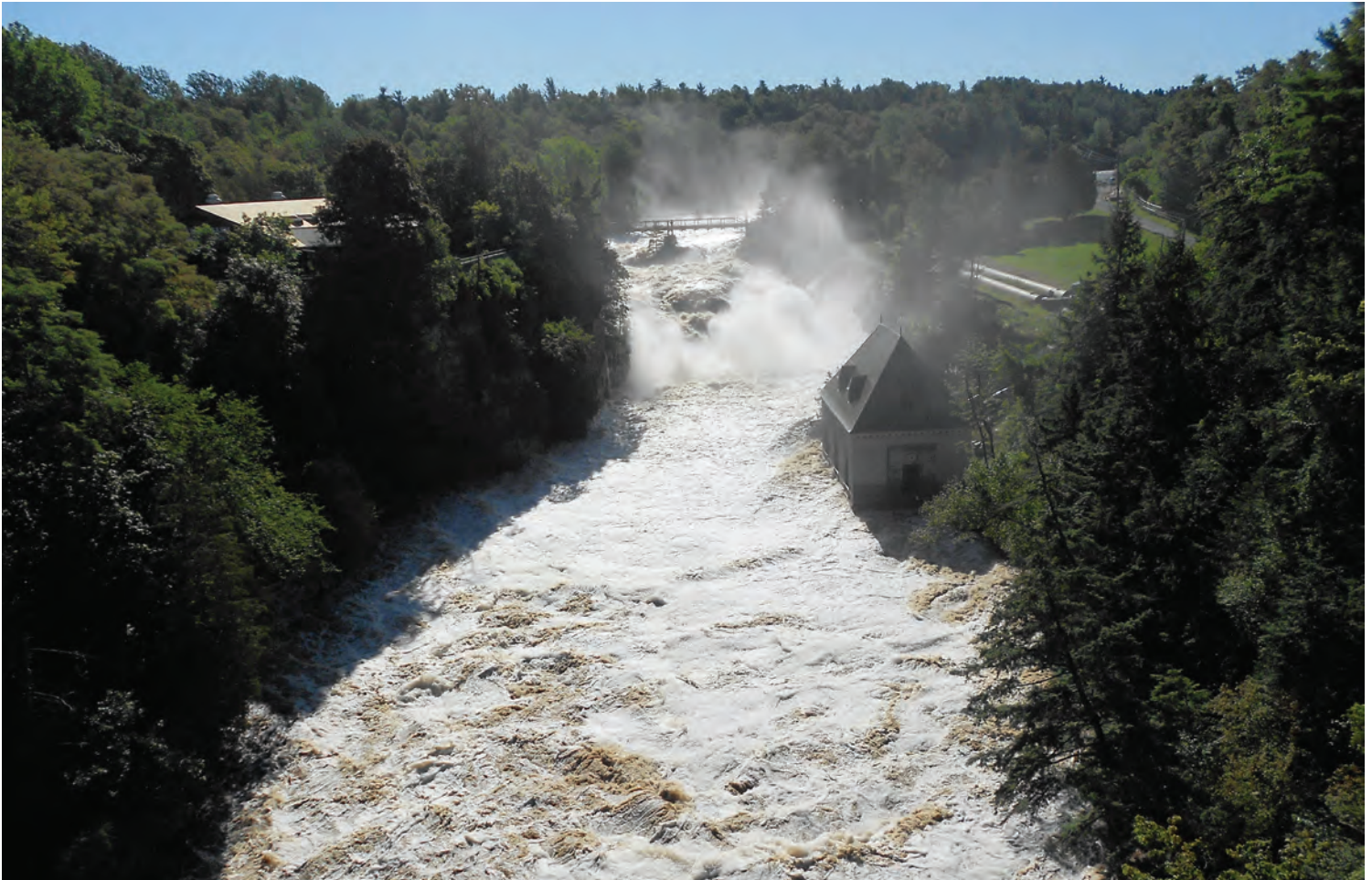
Hurricane Irene caused significant flooding to occur at NYSEG's Rainbow Falls Hydro Power Plant on the Ausable River.
