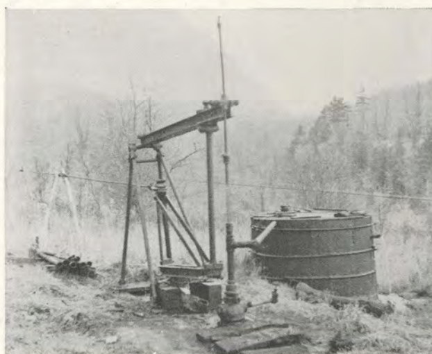
Oil pump with activating rod and water separation tank
