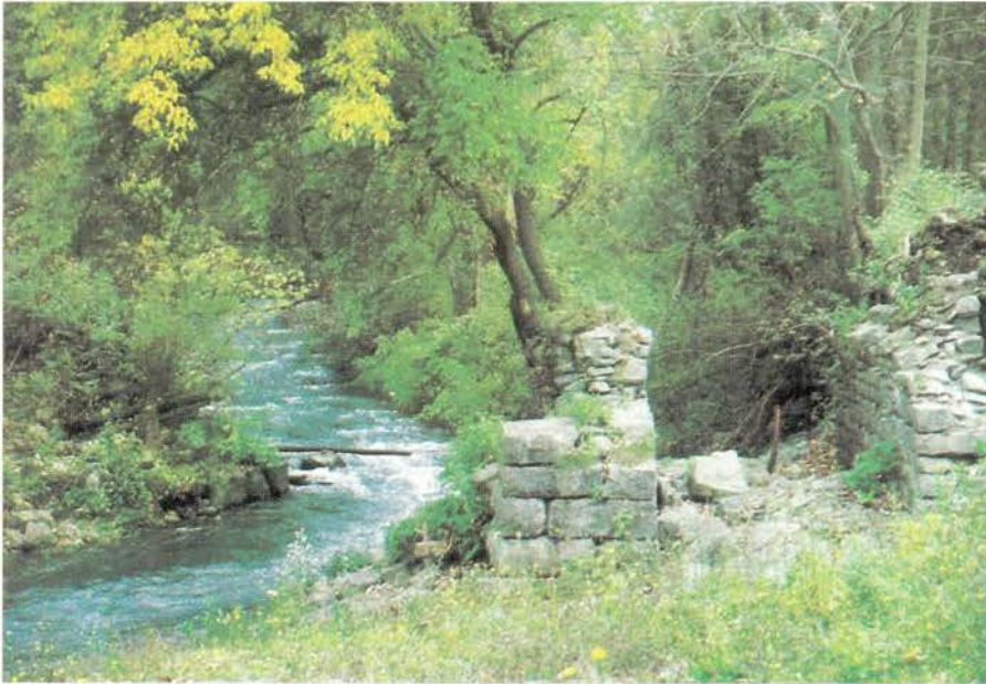
Morton's woolen mill at Mottville, one of 140 19th century factories on Skaneateles Creek, is now only a pile of foundation stones, a reminder of past uses.
