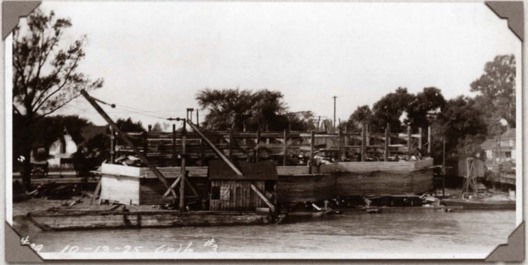
Construction of a wooden caisson along the Fort Erie shoreline in October 1925.
