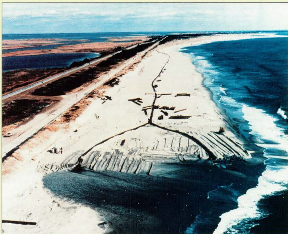
Beach nourishment project at Gilgo Beach, Jones Beach State Park, on the south shore of Long Island. Sand is dredged from the navigation channel in Fire Island Inlet (upper, right background) and pumped as a semi-liquid slurry through the 27-inch diameter pipeline on the beach. Roadway at left is Ocean Parkway which runs the length of Jones Beach Island, providing an emergency evacuation route.
