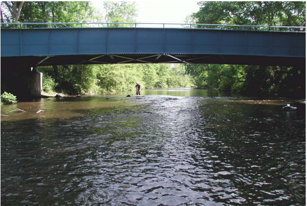
Figure 13-5. Wappinger Creek at Salt Point, 2002.
