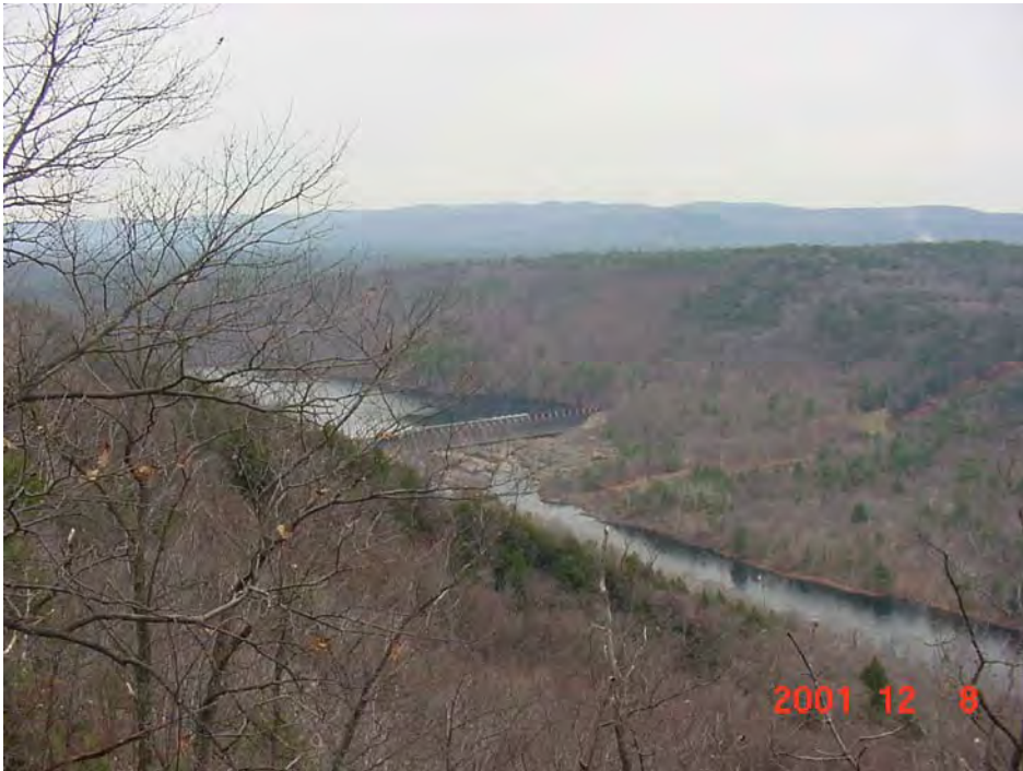
Western Ridge Trail, central, spur 2 dam
