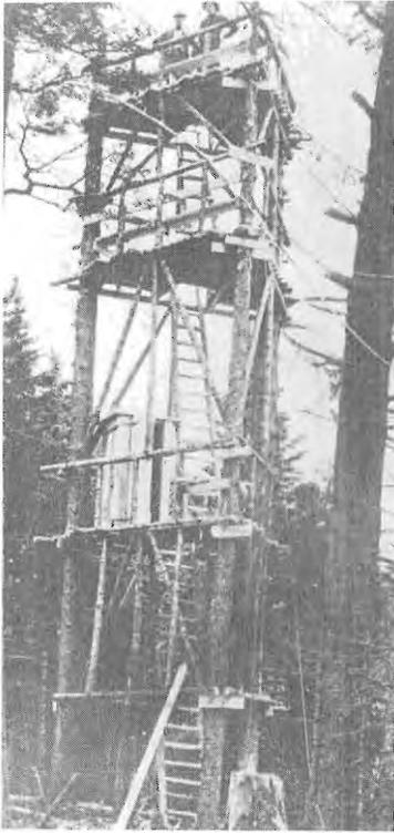
*Early fire observation stations were equipped with crude log or plank towers.*
