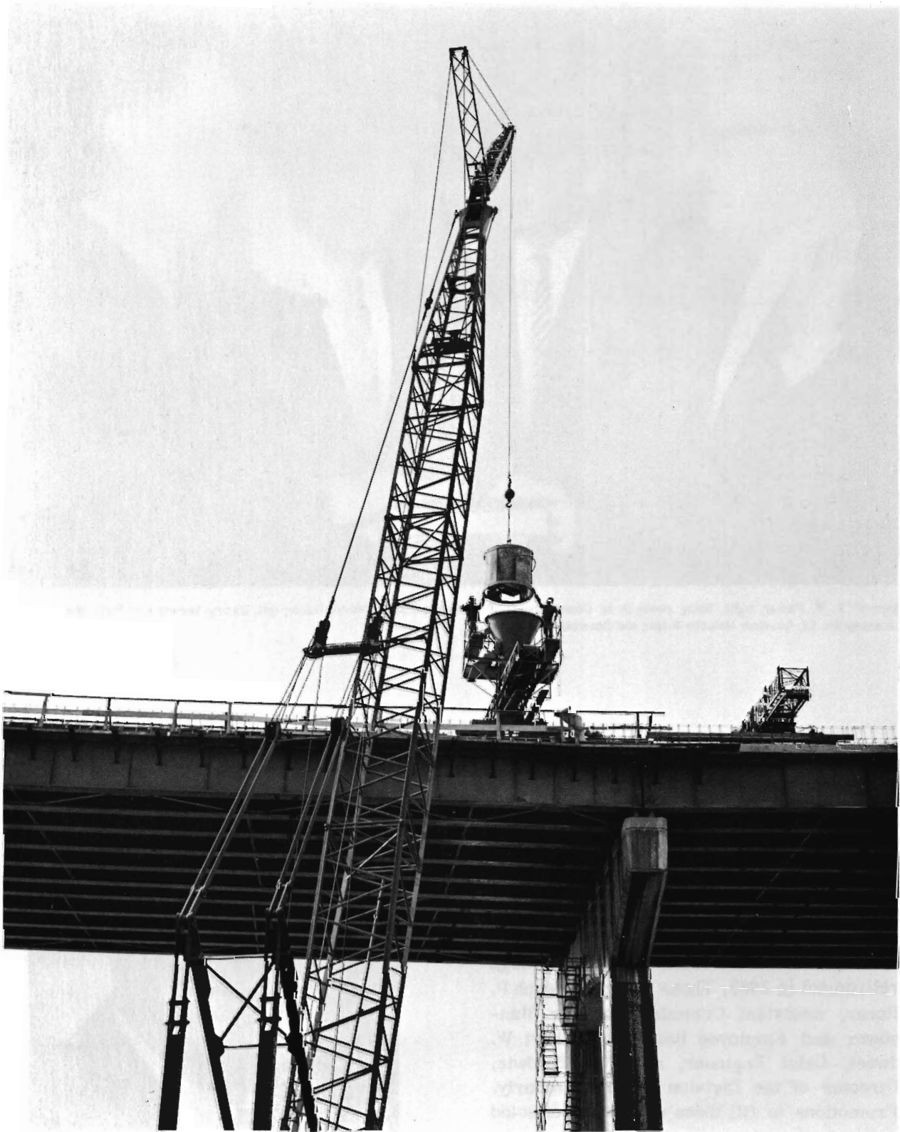
Bridge approach construction for Albany's arterial highway system.
