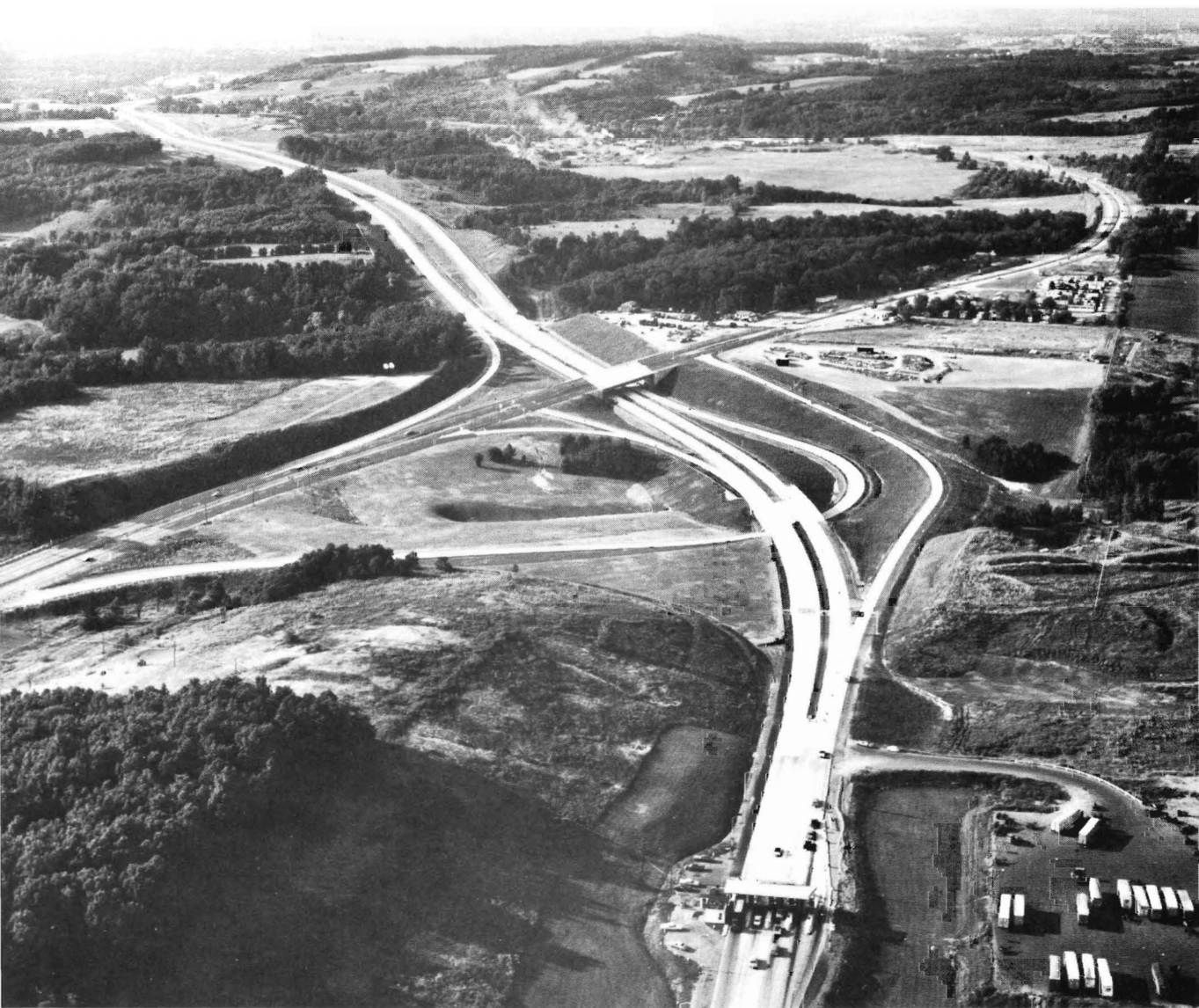
This section of the Eastern Expressway (Interstate Route 490) was opened to traffic in 1969. It completes the route which now extends from the Governor Thomas E. Dewey Thruway near Victor to Rochester. Thruway toll booths can be seen in foreground.
