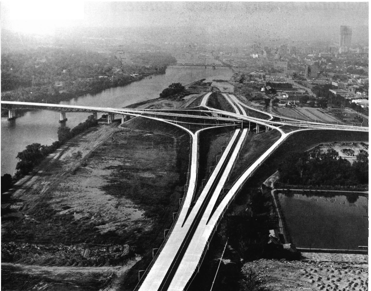
The new Patroon Island Bridge at Albany. Pavement in foreground is part of uncompleted Albany Riverfront Route (Interstate Route 787).
