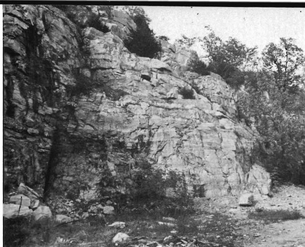
Figure 62. Warner Hill Limestone Member of Whitehall Formation; abandoned quarry on north side of Washington County 10, 2 miles northeast of Whitehall.
