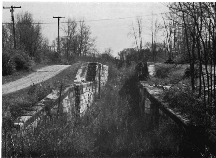
Figure 11. Abandoned lock on former Champlain Canal; east edge of village of Fort Ann. Dimension stone constructed of various Beekmantown carbonates and Isle la Motte Limestone.
