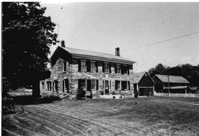
Figure 58. Private home constructed of Potsdam Sandstone dimension stone, 3.8 miles east-northeast of Fort Ann, Dewey Bridge Road.
