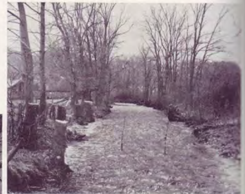
An improved stretch of the Little Hoosick showing stumps of potential stream blockers which were removed to keep them from falling into and eventually blocking the stream. The less debris, the faster the flow and the less the erosion damage.
