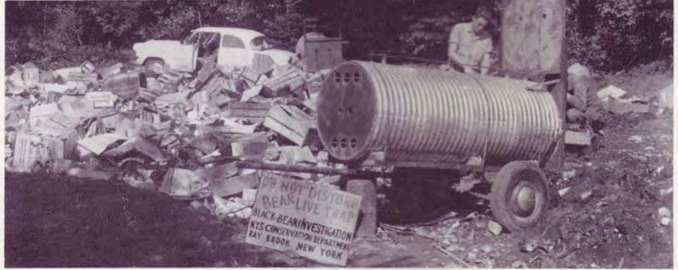
Live-traps are trailer-mounted culvert sections.
