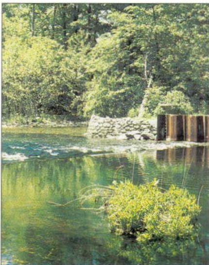
(Above) Weir across the Bashakill Creek in Sullivan County replaces a natural gravel bar that was subject to washouts during periodic flooding.
